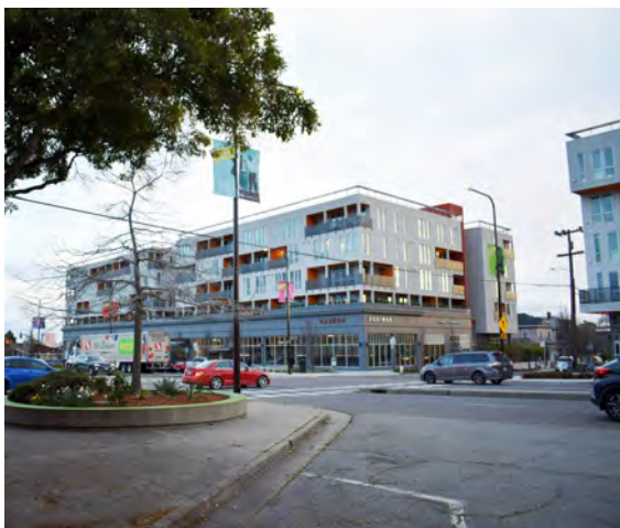
Existing mixed-use building in the South Shattuck subarea
