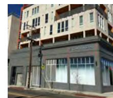
New development preserves the historic storefront facade
